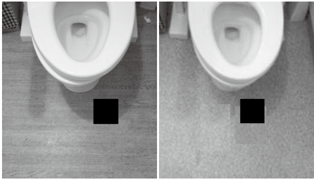
1) Before construction 2) After construction Fig.6 Photos showing measurement point in toilet floor.
